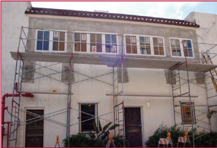
Impact-resistant windows are now installed.
